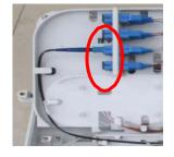
3. Install the 1x8 or 1x16 splitter in the location shown below
