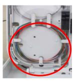
8. Installed the connectors from the drop cables into the bulkhead connector of drop cable
